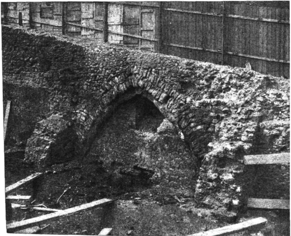
ARCH NO. 1, UNDER CASTLE BRIDGE.
